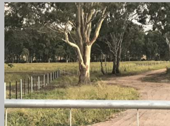
Construction of fencing
