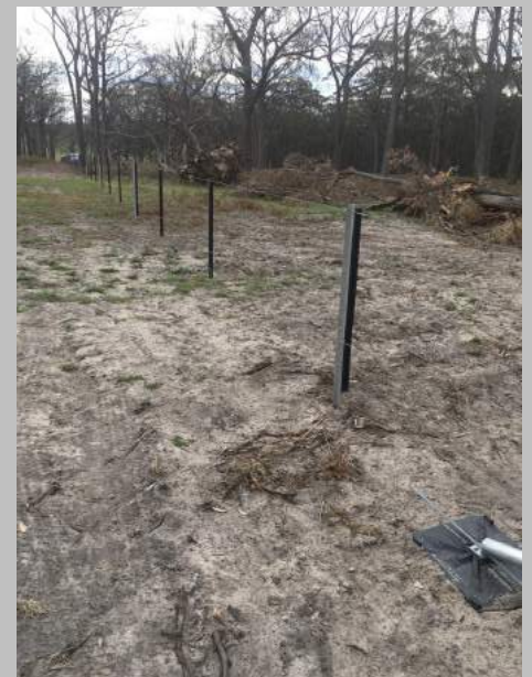
Fencing is constructed to allow grazing management change
