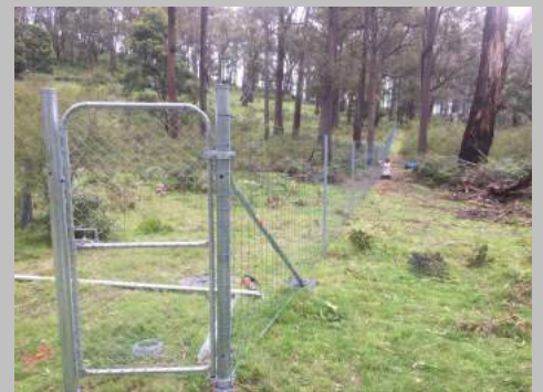
Construction of deer exclusion fencing
